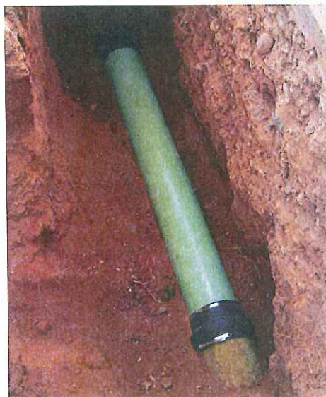
Figure 14 - Point Repair
