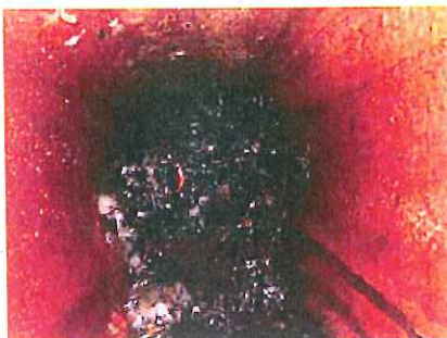
Figure 8 - Root Ball Barrell (RBB) Defect
