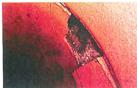
Figure 3 - Broken Soil Visible (BSV) Defect
