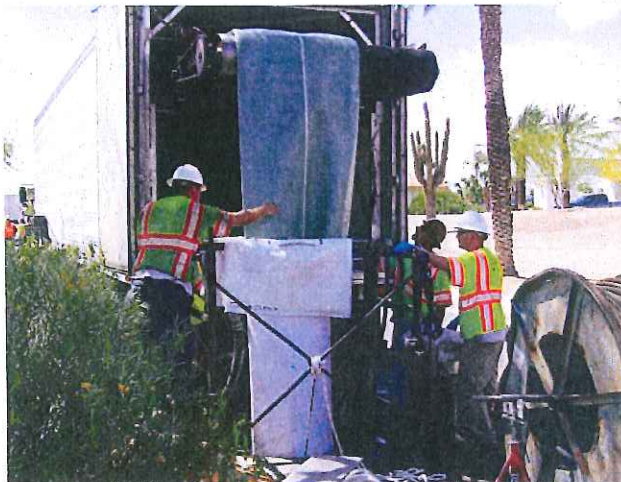
Figure 15 – Inversion CIPP Liner Insertion
