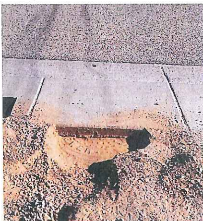
Figure 1 – Calle Batoua Buried Manhole
