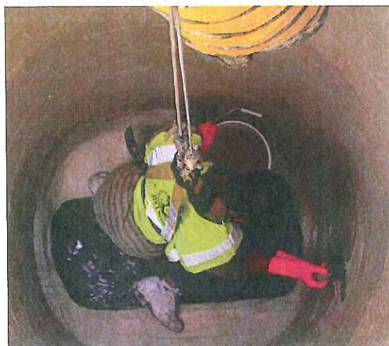
Figure 10 – Trowel Epoxy Coating Application
