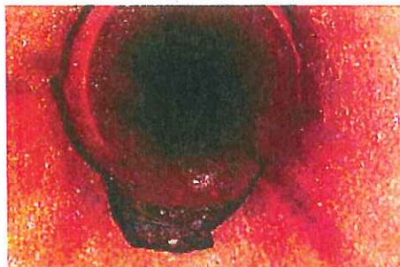
Figure 4 - Hole Soil Visible (HSV) Defect
