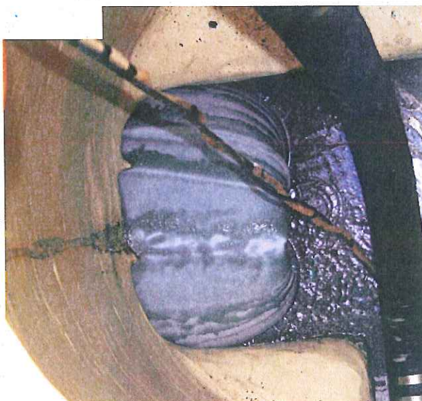
Figure 16 – Inflated CIPP Liner at Manhole Invert
