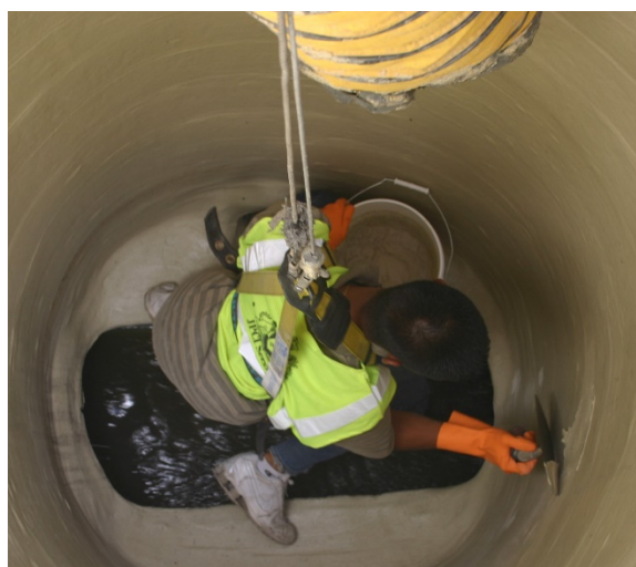
Figure 13 – Trowel Epoxy Coating Application
