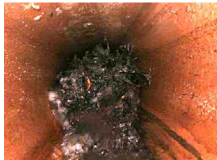
Figure 7 - Root Ball Barrell (RBB) Defect
