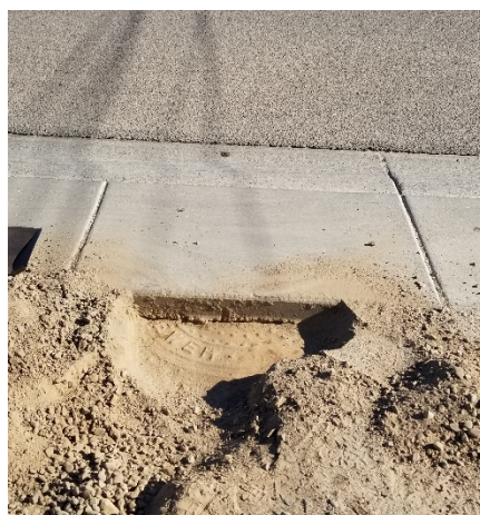
Figure 9 - Buried Manhole
