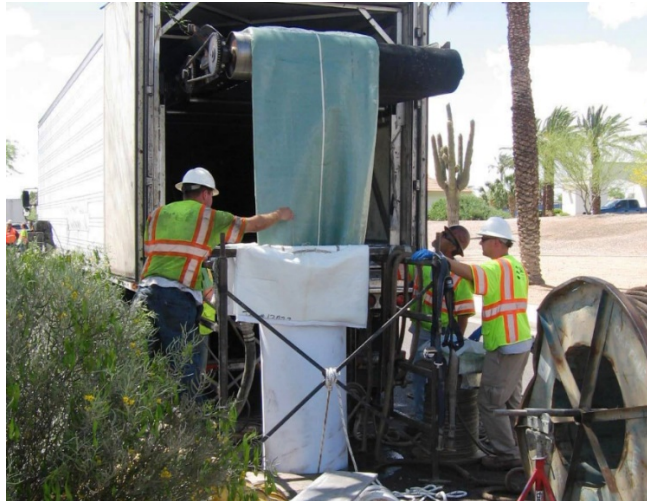
Figure 11 – Inversion CIPP Liner Insertion
