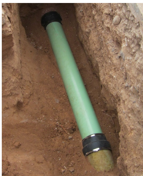
Figure 10 - Point Repair
