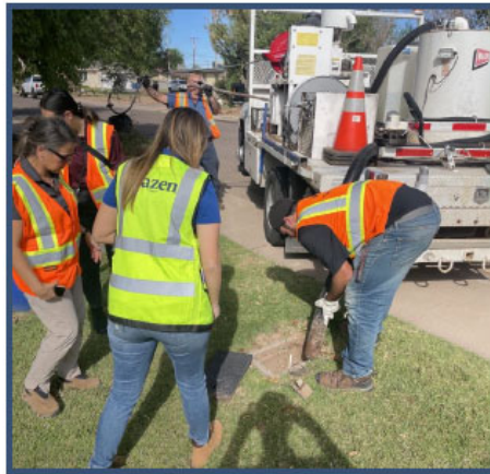
Inside Meter Box Excavation (Tier 1)
