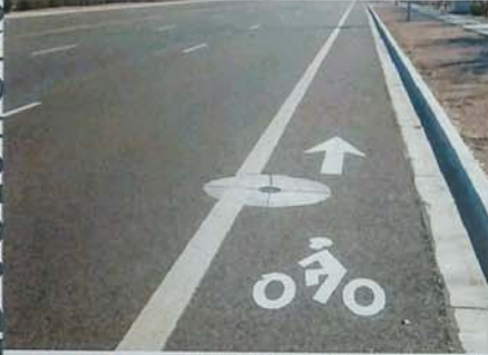
BIKE LANE + CURB AND GUTTER
