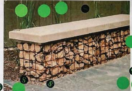
GABION SEAT WALL
