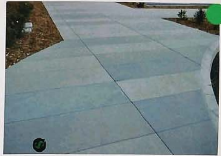
DECORATIVE CONCRETE JOINTS
