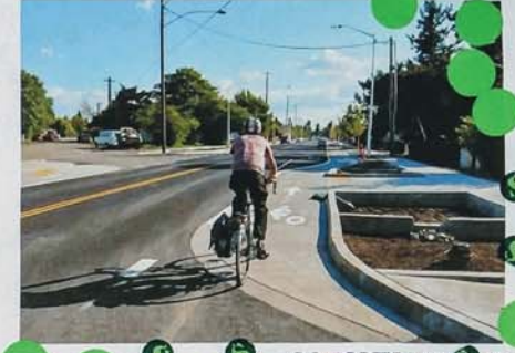
CONCRETE BIKE LANE
