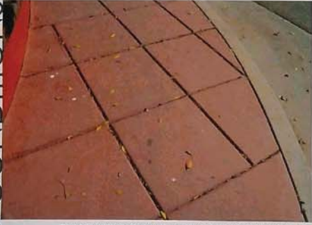
EXISTING SIDEWALK EXPANSION JOINTS
